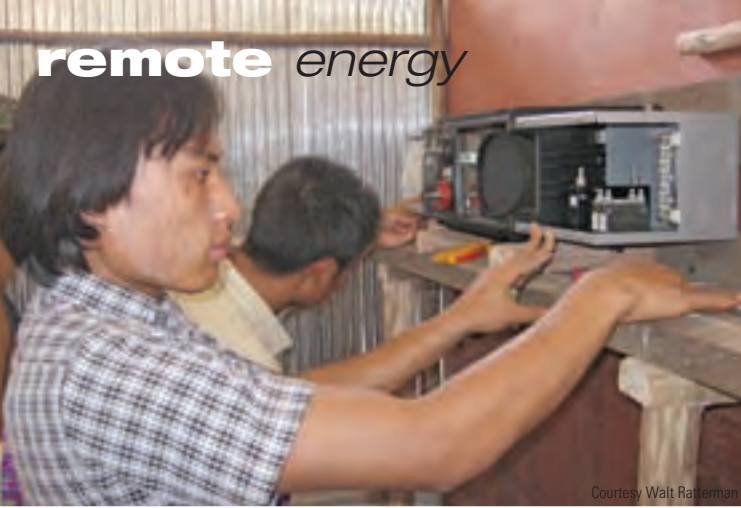
Refugees at a camp on the Thailand–Burmese border install an inverter and charge controller.
